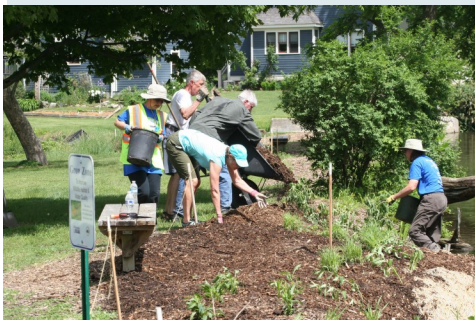
Volunteers stabilize the eroding streambank with coir logs and plant a buffer of native wildflowers, shrubs and grasses at the Historic Mill Race Village work site
