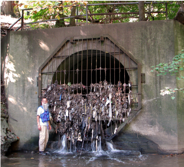
Volunteer standing next to a combined sewer overflow outfall
