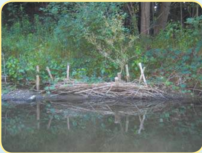
Figure 48 - Log matrix used to armor bank
