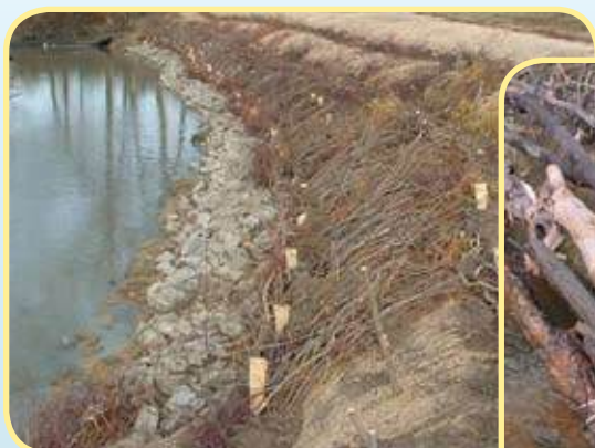
Figure 55 - Woody debris and rip rap combined to armor a streambank
