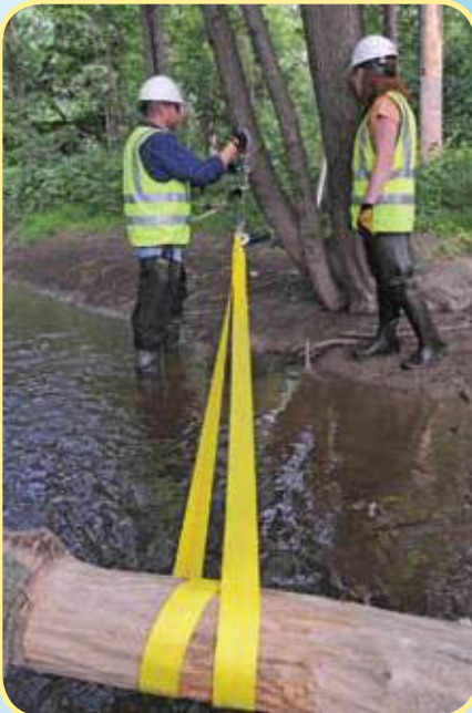
Figure 29 - Using a come-along to reposition log
