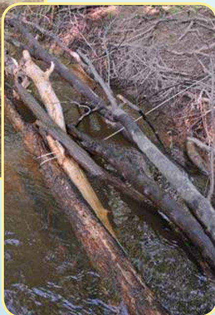
Figure 56 - Logs cabled together to armor eroding bank
