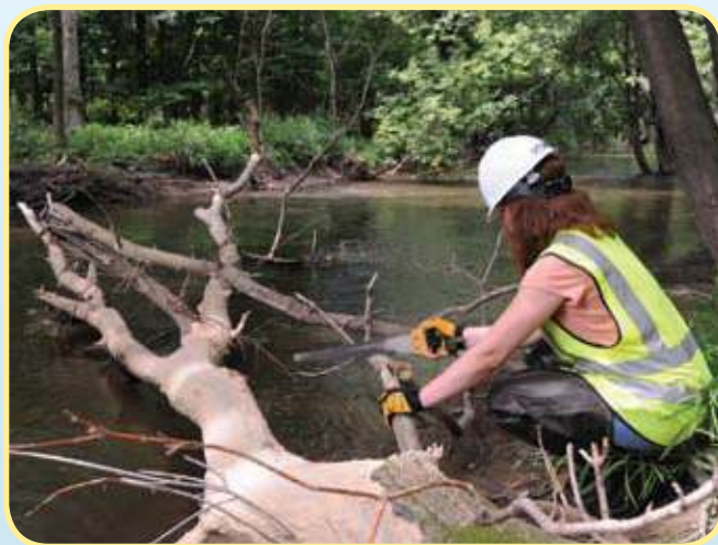
Figure 10 - Using hand tools for LWD maintenance
