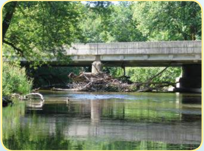
Figure 42 - LWD blocking culvert
