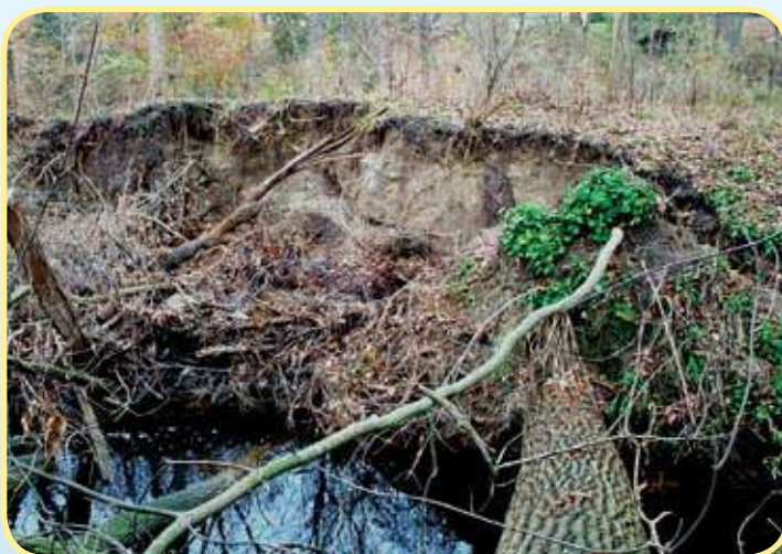
Figure 59 - LWD structure causing bank erosion
