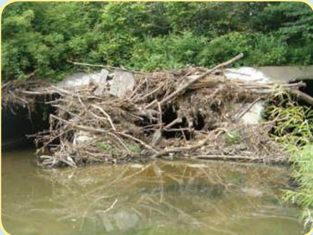
Figure 42 - LWD blocking culvert
