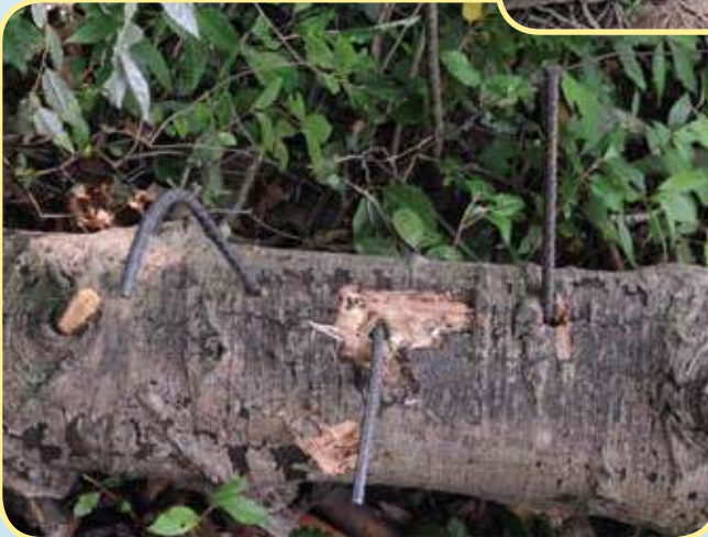
Figure 33 - Bend rebar to secure log in place. The easiest way to bend rebar is to apply leverage to the top of the bar after it has been pounded into the woody debris and substrate.
