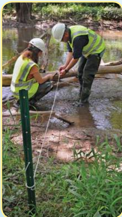
Figure 50 - Anchoring a log using the Palmiter Method
