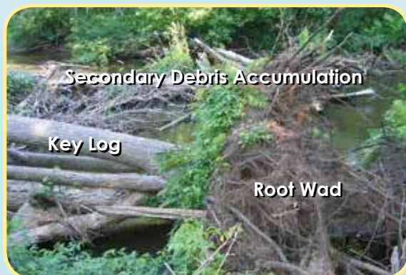
Figure 2 - Typical components of a LWD structure including the key log, root wad, and secondary debris accumulation
