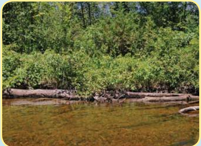
Figure 6 - LWD armoring stream bank
