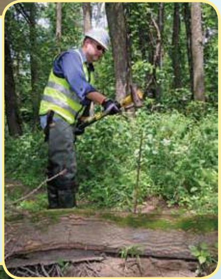
Figure 32 - Anchoring log to bank with rebar
