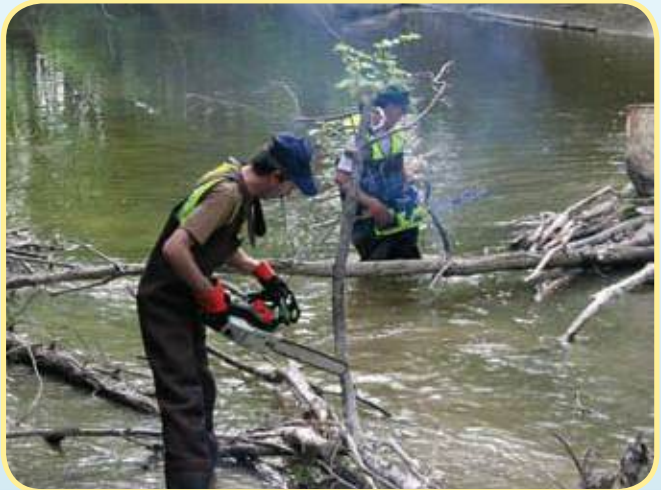
Figure 22 - Placing cut debris above bankfull channel
